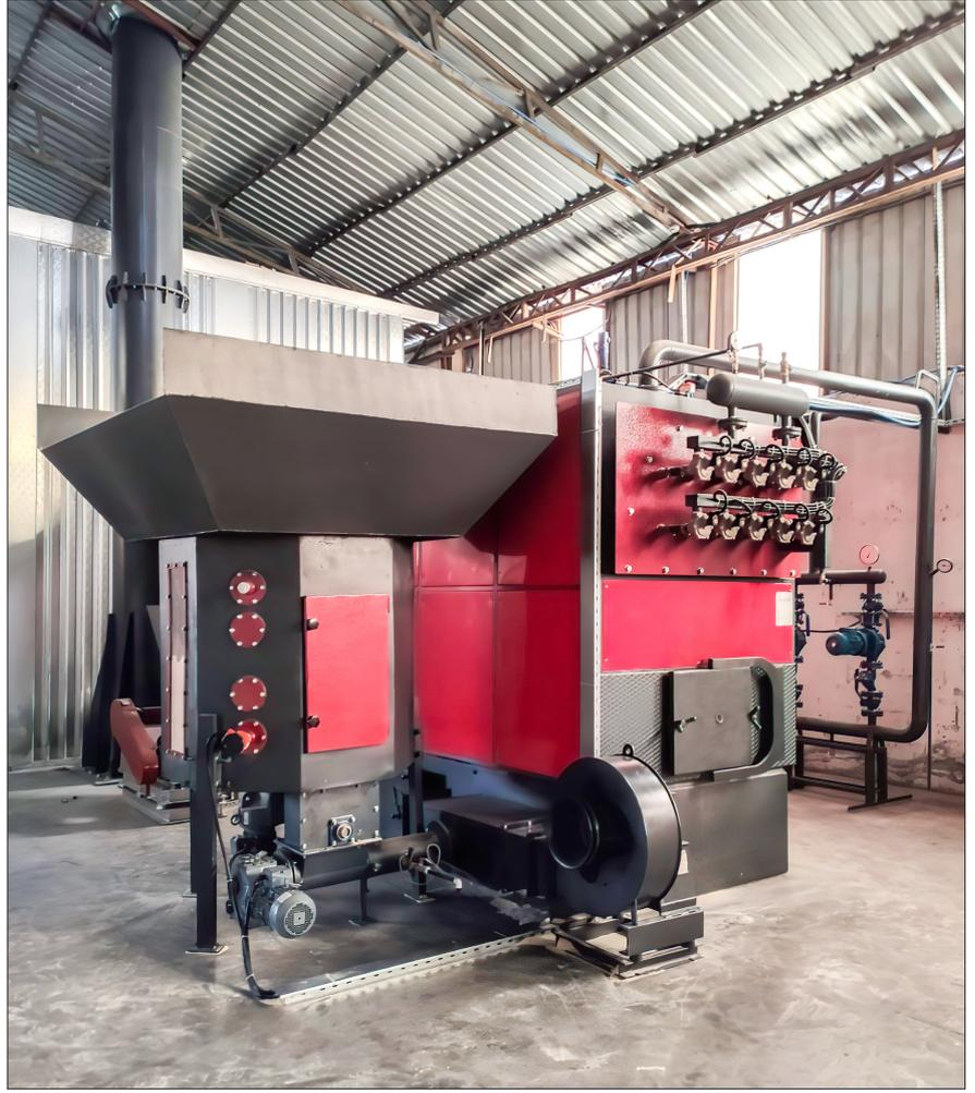
With biomass boilers, cheap and safe energy (hot water, superheated water, hot oil, steam) is obtained from factory wastes that have no economic value which are released as a result of manufacturing in your business such as pieces of wood, wood chips, MDF powder and paper.
