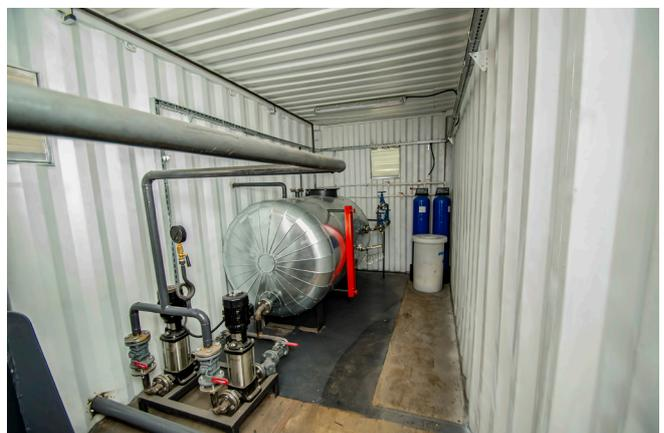
As all plumbing connections come from a single point, it is very practical to use, install and maintain. The structure of the unit very robust, functional, compact, long-lasting and made to fit the equipment used. The front cover is manufactured in a way that can be opened completely, and it is simple to maintain and repair.
