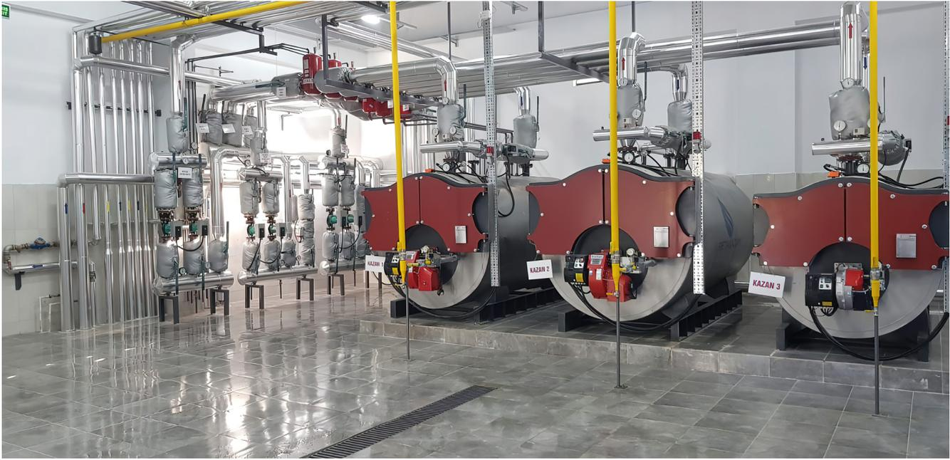
It is produced with computer aided design and high manufacturing technology in accordance with production standards, PED pressure vessels directive, TS EN303-1, TS EN12953 standards.
