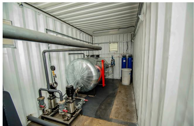
As all plumbing connections come from a single point, it is very practical to use, install and maintain. The structure of the unit very robust, functional, compact, long-lasting and made to fit the equipment used. The front cover is manufactured in a way that can be opened completely, and it is simple to maintain and repair.
