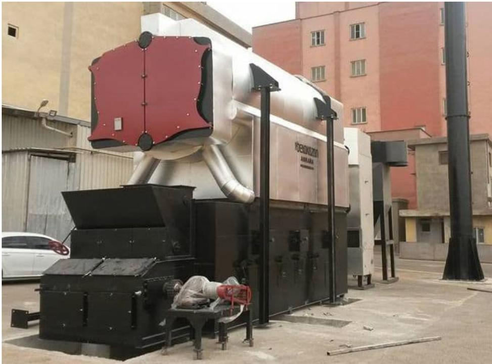
It is a combustion unit with a conveyor grate mounted under the water pipe primary combustion chamber.
